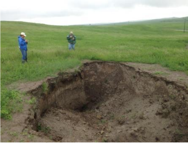
This picture, taken June 11, 2014, shows a dangerous sinkhole at the Haynes site, near the South Dakota border. It was about 30 feet long, 15 feet wide and 10 feet deep.
