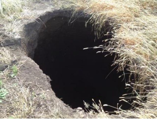
This sinkhole was on a farm trail on Garner Sailer's property located about 2 miles northeast of Beulah. It was over 20 feet deep and a hunter dropped the front wheel of his Suburban into it.
