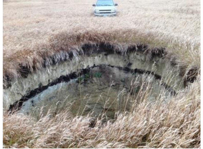
This shows another sinkhole at Garrison, about 18 feet across and 12 feet deep. Note the coal stringer 3-4 feet below surface. These sinkholes were close to businesses on the south side of Garrison.
