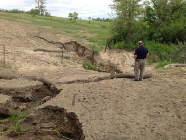
This shows erosion leading to a large sinkhole on property owned by Dave Zimmerman, near Richardton. This was the site where a large sinkhole was filled in 2013.
