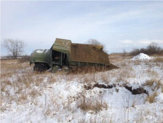
This sinkhole, on Jim Krzmarzick's pasture, was found when the back wheel of a loaded truck dropped into it.
