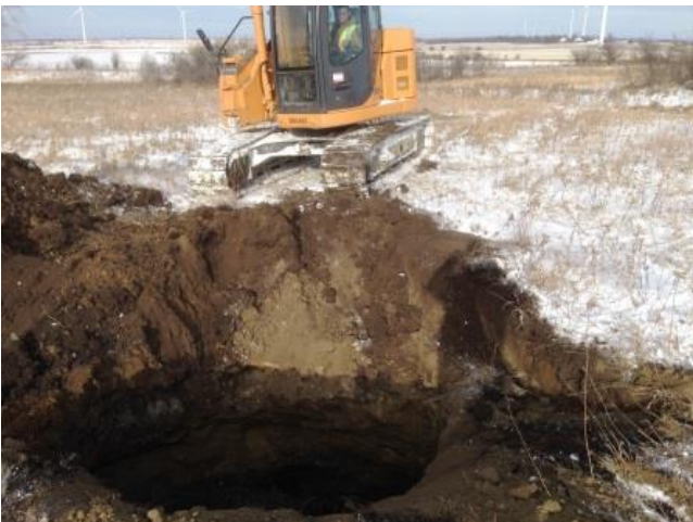
This is the same hole after the truck was pulled out and topsoil was removed. It was about 12 feet across and 10 feet deep. No one was injured and the truck was not damaged. A close call.
