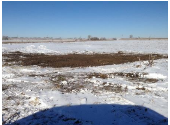
This was the last sinkhole filled in the project on a cropland field owned by Betty McGinnis. Seventy-four sinkholes were filled at the Wilton Site between November 6 and 14. The cost was $17,070.
