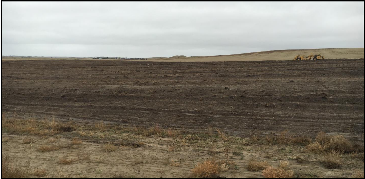
Top: Final grade of the north site
