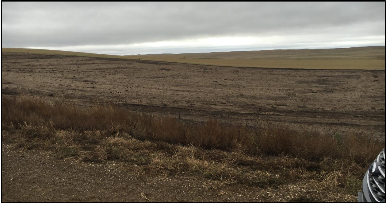
Bottom: Final grade of the south site
