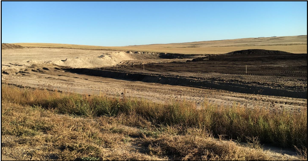
Bottom: Partial completion of filling the pit of the south site
