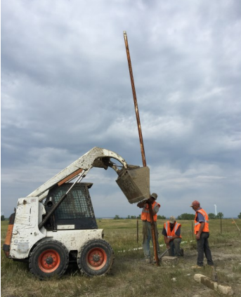
Removing casing from filled hole.
