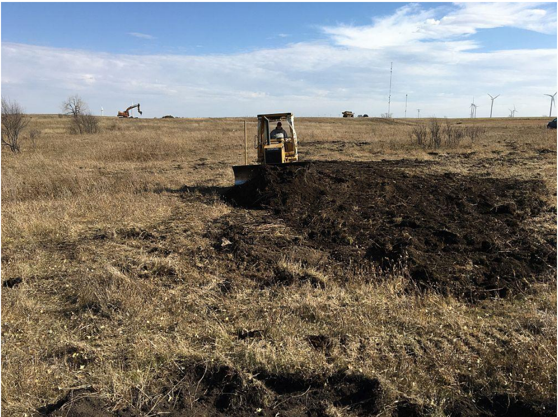
This shows a dozer spreading topsoil over a reclaimed sinkhole at the Wilton Site prior to tilling and seeding. The approximate cost of sinkhole filling at Wilton was $9977.50.
