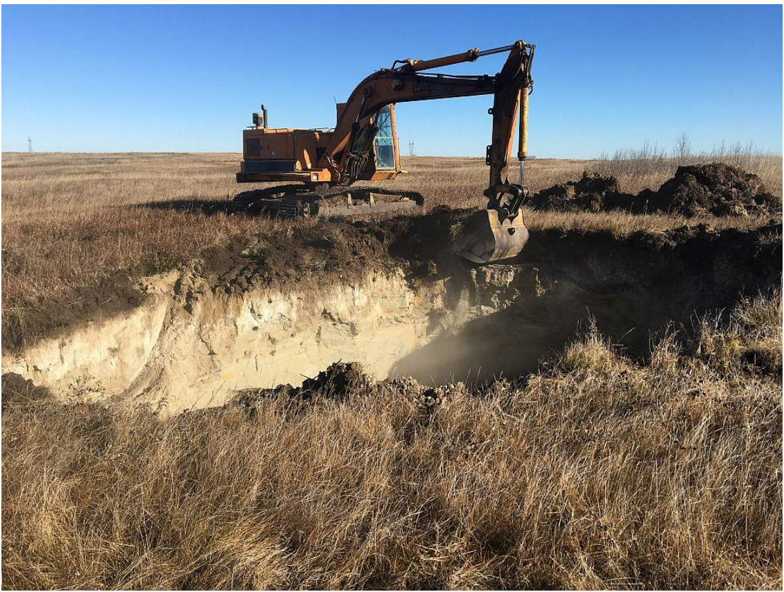
Approximately 23 dangerous sinkholes were filled October 26 through November 8 on North Dakota Game and Fish property north of Beulah. The contractor was saving topsoil from a sinkhole that was about 25 feet long, 20 feet wide and 20 feet deep.
