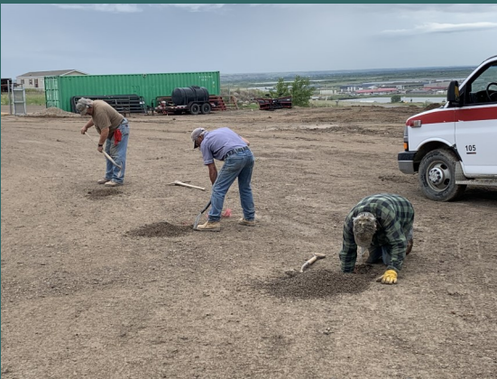
Left: Contracting crew locating cased holes for pumping grout in Williston.
