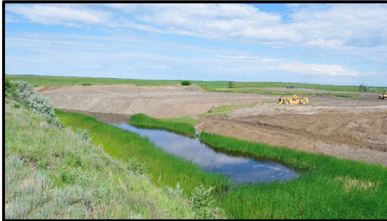
Photo 3 - Contractor backfilling the Southeast pit (looking northwest)
