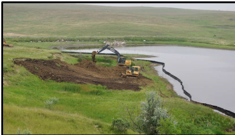
Photo 6 - Contractor backfilling the highwall on the East Site
