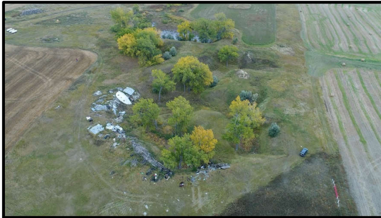
Photo 18 - Timpe pre-reclamation (looking east)
