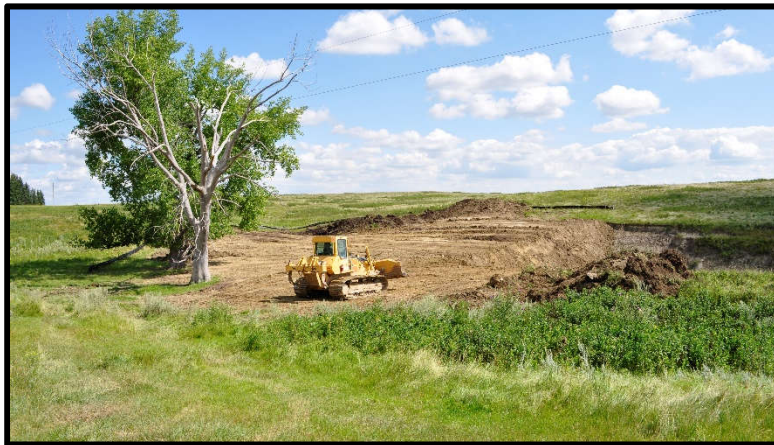
Photo 17 - Contractor backfilling the highwall
