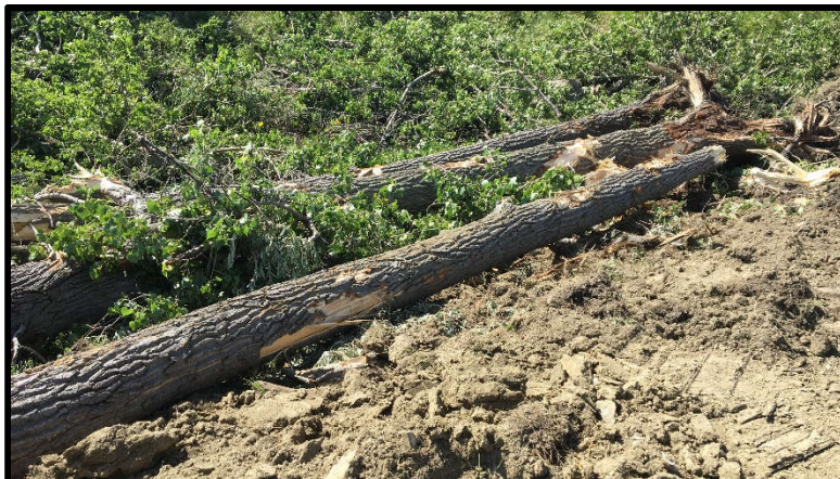
Photo 19 - Some trees that were felled by the contractor
