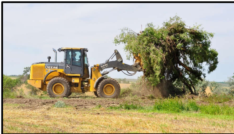
Photo 15 - David Doll, property owner, piling trees on site
