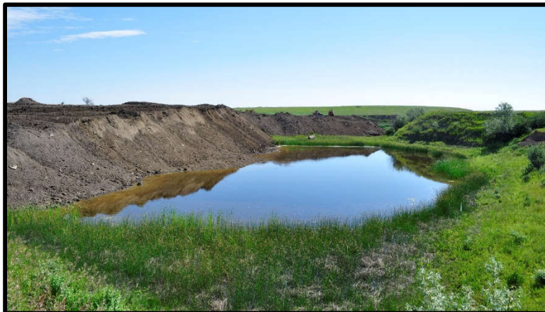
Photo 4 - Contractor backfilling the Southwest pit (looking northeast)
