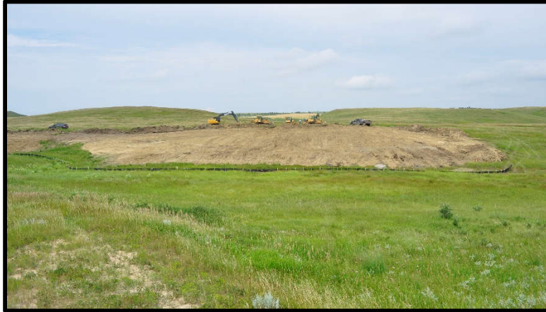
Photo 10 - Contractor backfilling the pit at the West Site
