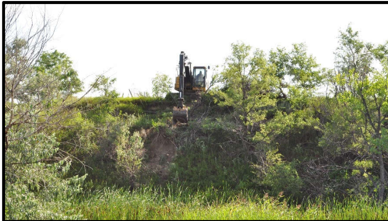
Photo 13 - Contractor clearing trees from the highwall
