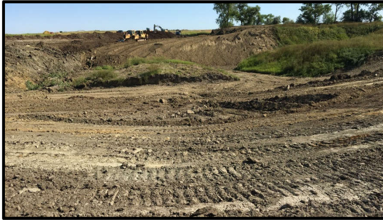
Photo 20 - Contractor moving dirt to the pit
