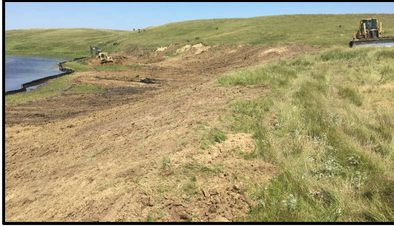
Photo 7 - Contractor backfilling the highwall on the East Site
