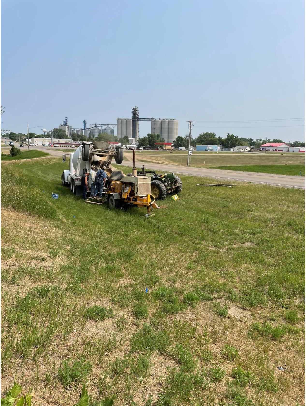
Figure 3: Grout is being pumped in the ditch of McLean County Highway 15.
