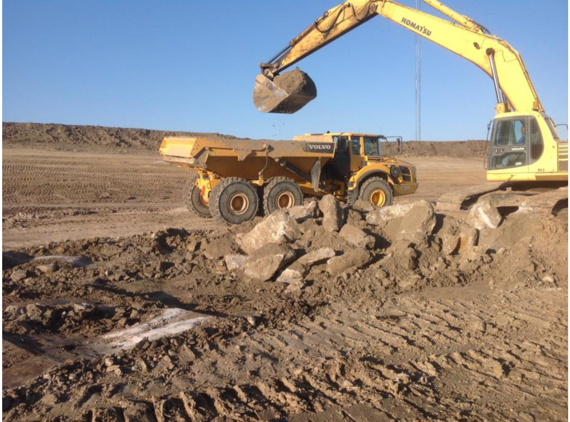
Excavator and Truck Utilized to Move Rock
