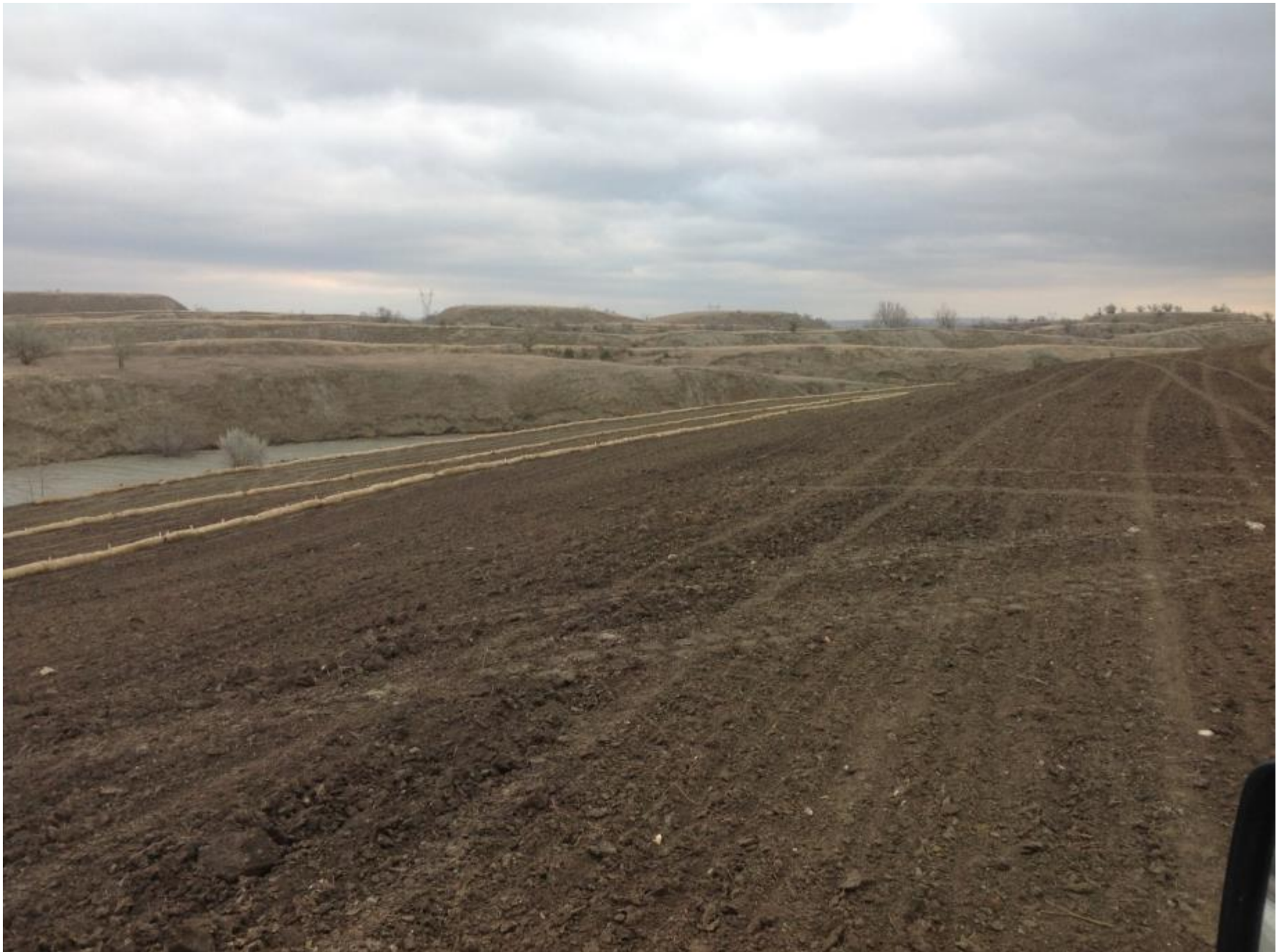
Straw Wattles Established
