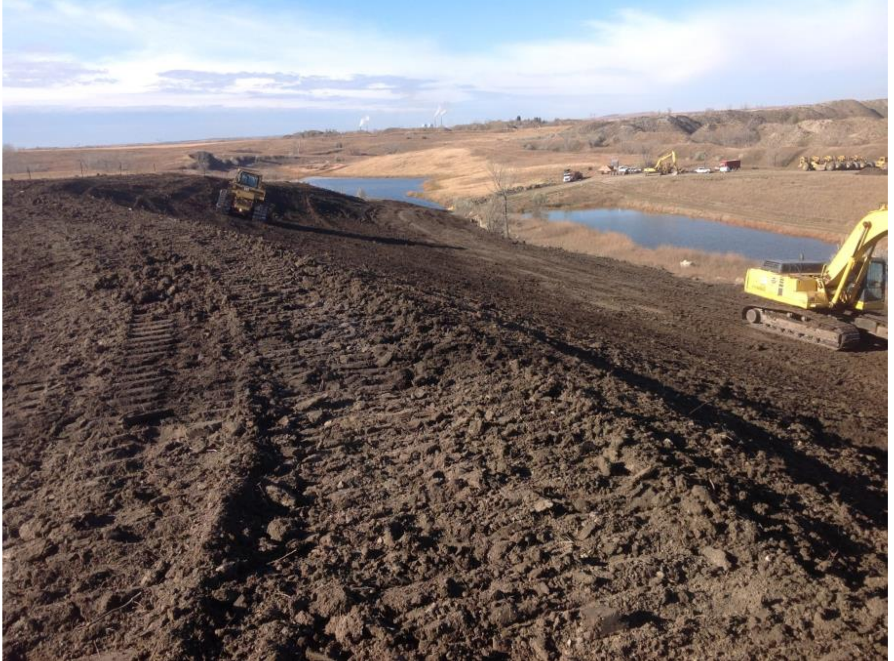
Dozer Leveling Respread Topsoil
