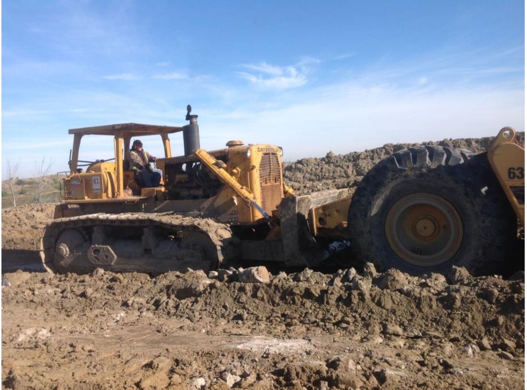
D9 Dozer Push Loading 631 Scraper
