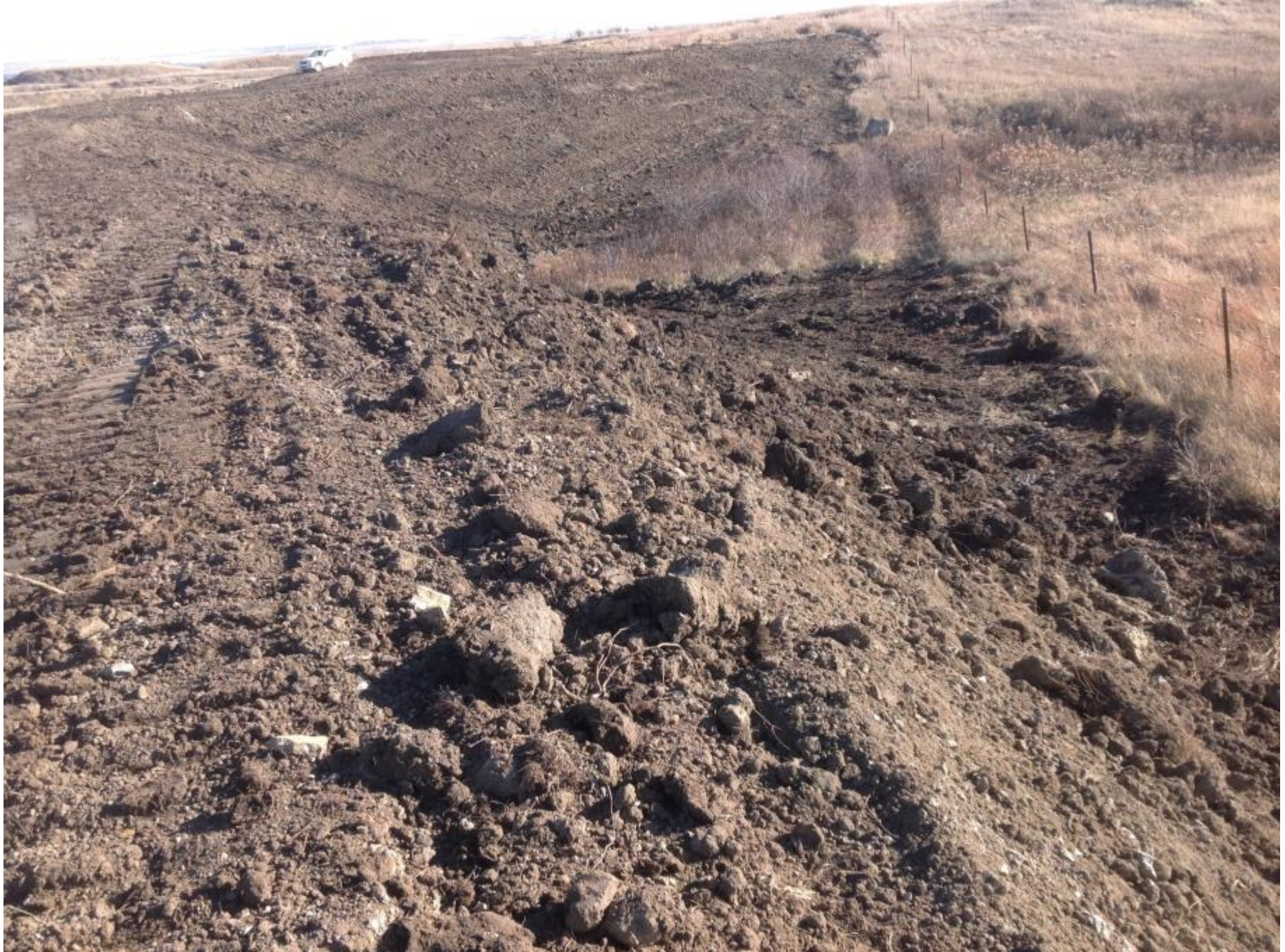
Embankment Established to Create Wetland Pond Needed to Control Surface Water Runoff
