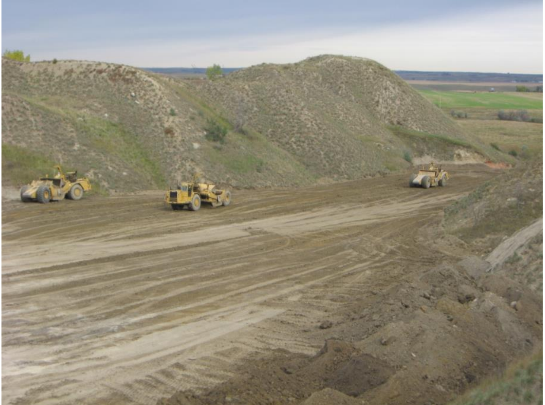
631 Scrapers Unloading in the Project Fill Area
