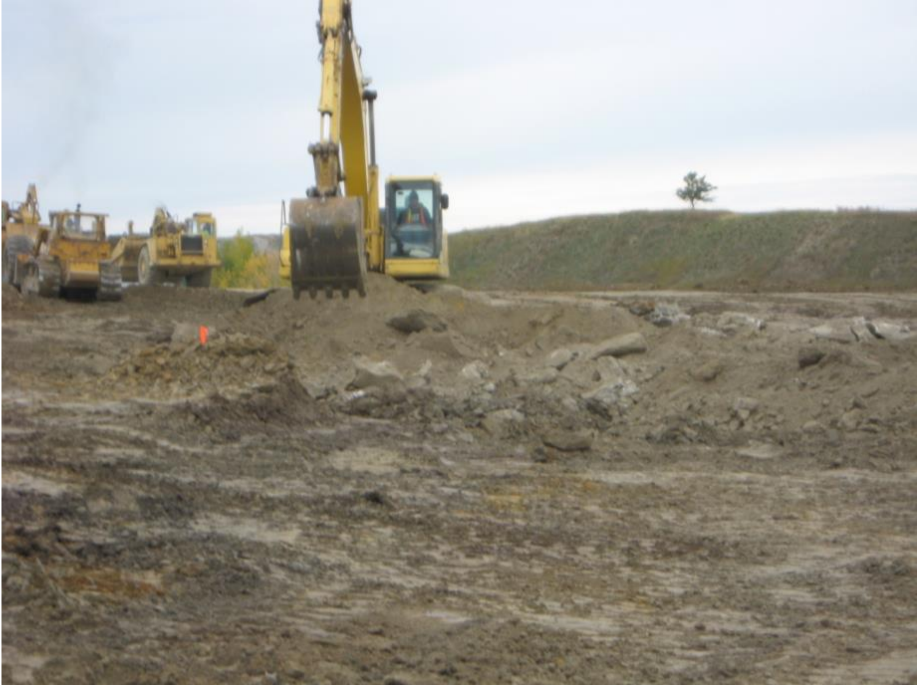
Contractor Utilizing Excavator to Digging Up Rock On-Site
