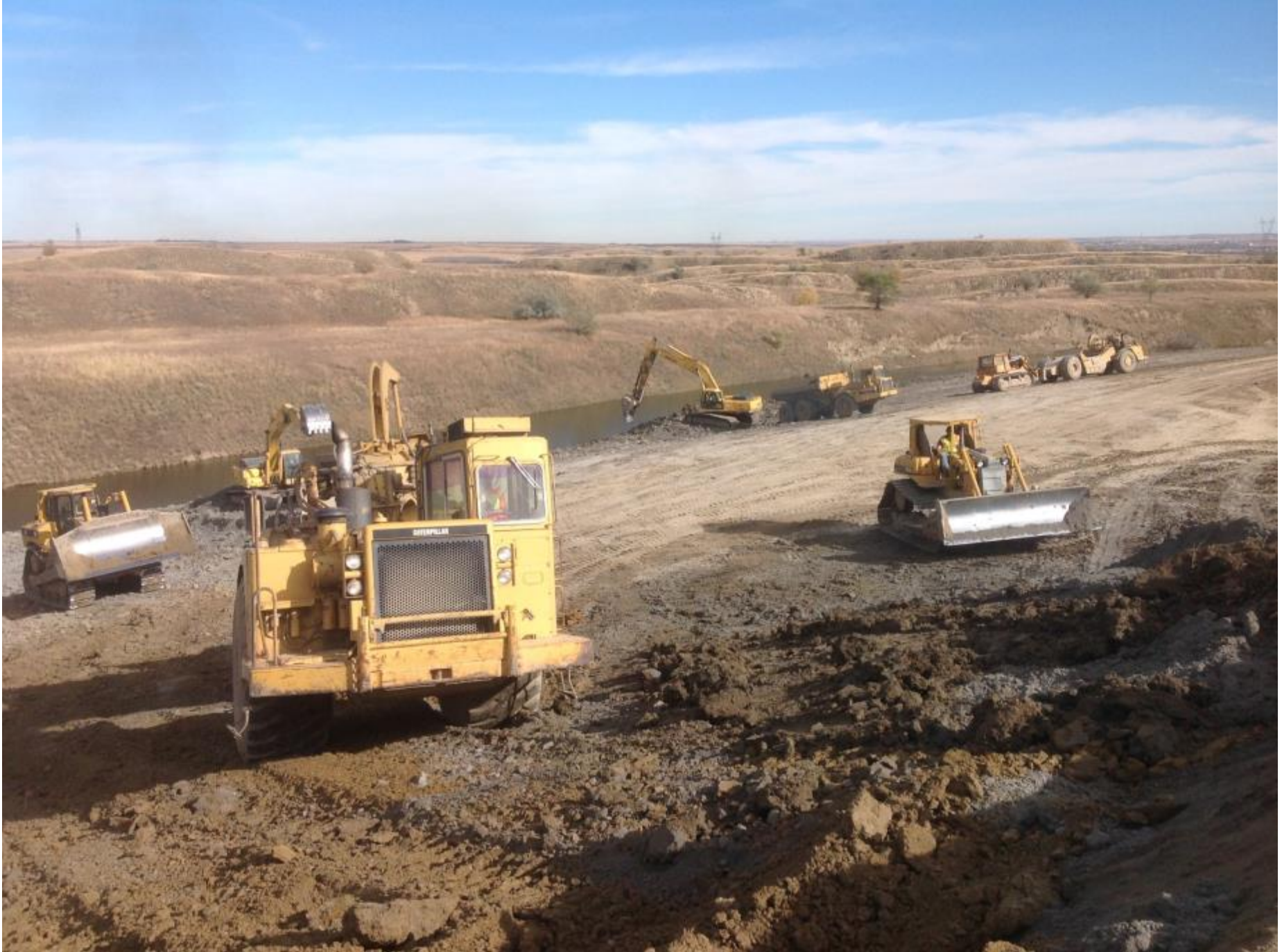
Construction Equipment being Utilized During Reclamation
