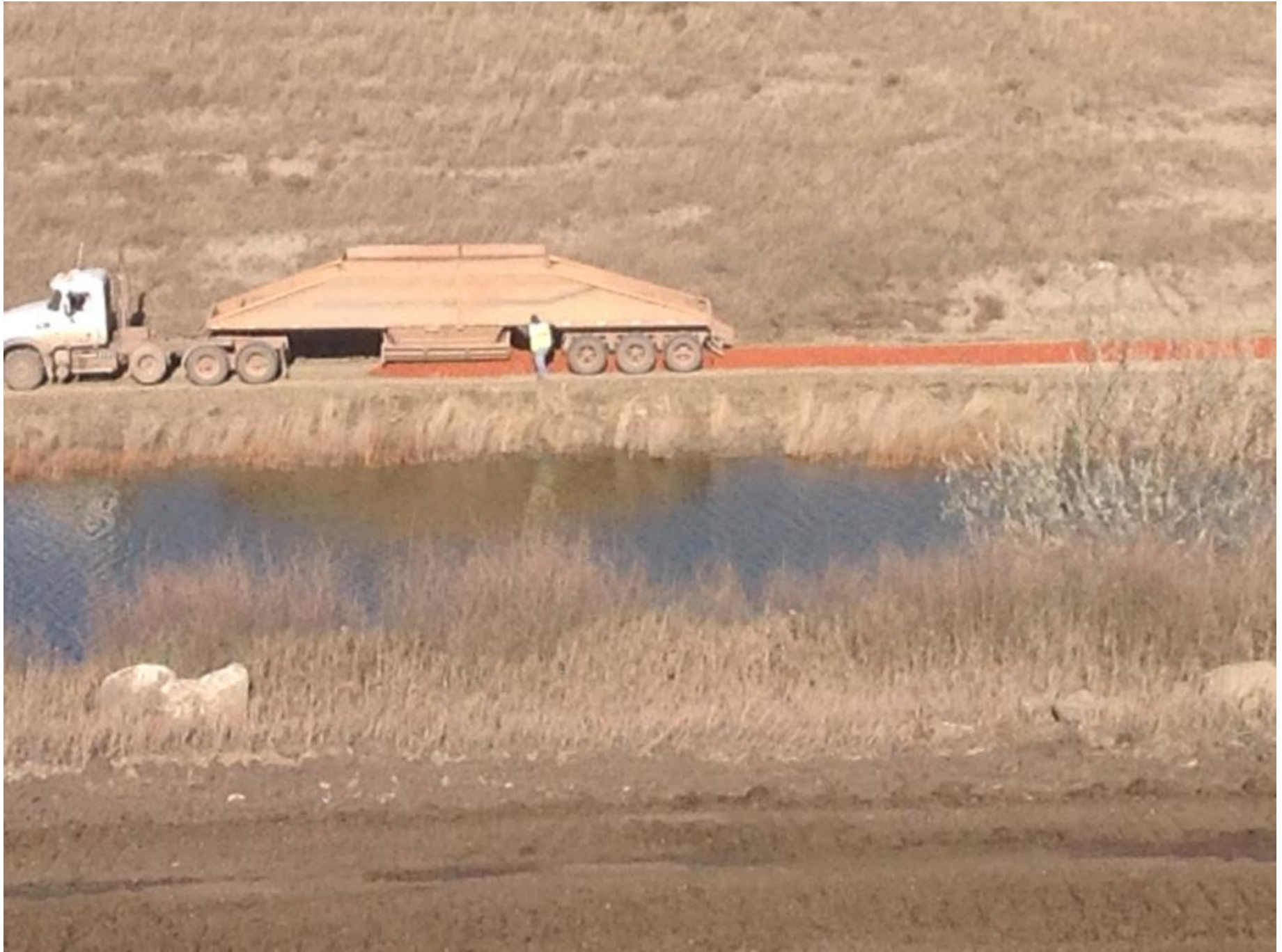
Scoria being placed along Shoreline of Bass Pond
