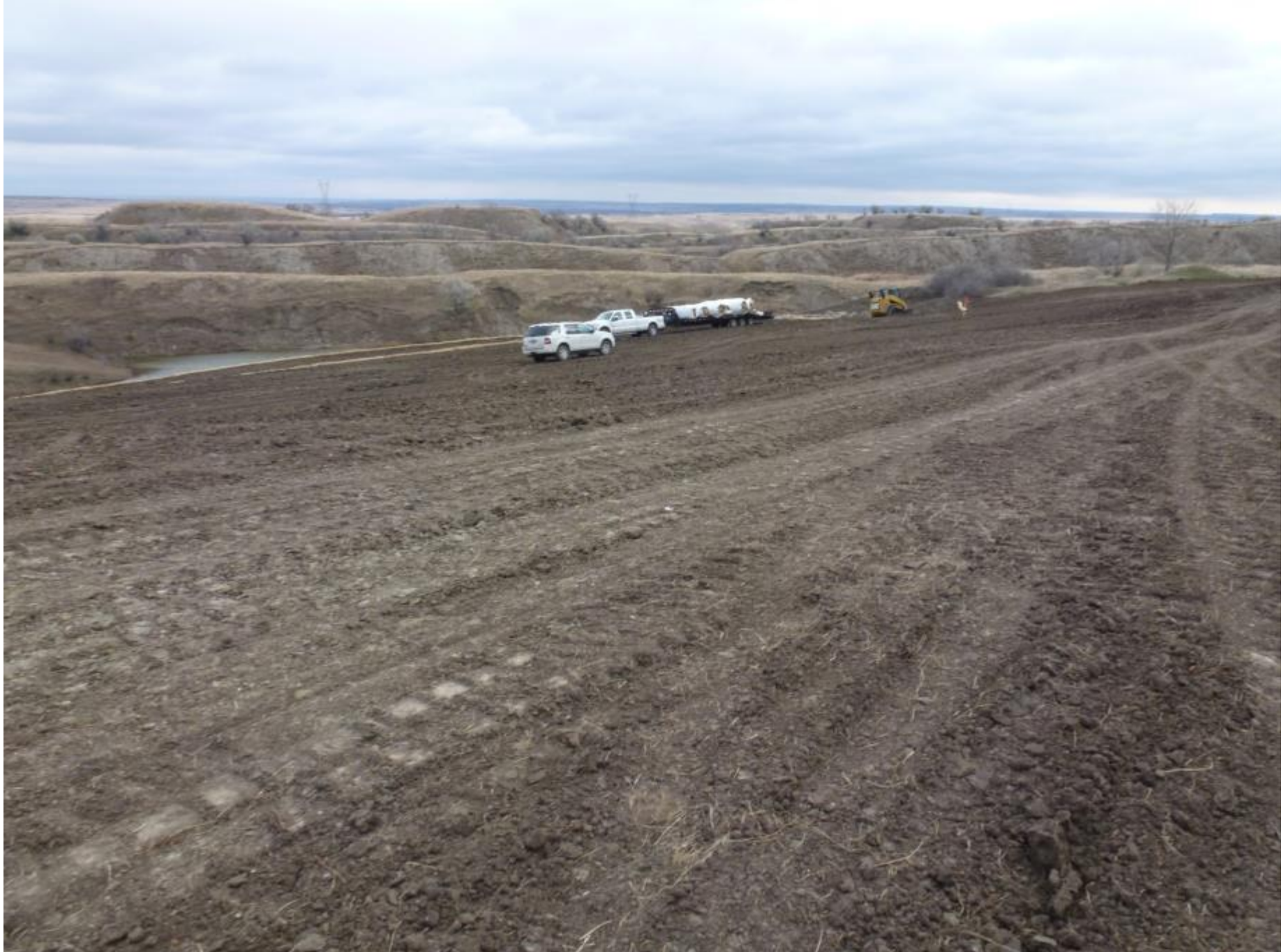
Placement of Straw Wattles for Erosion Control
