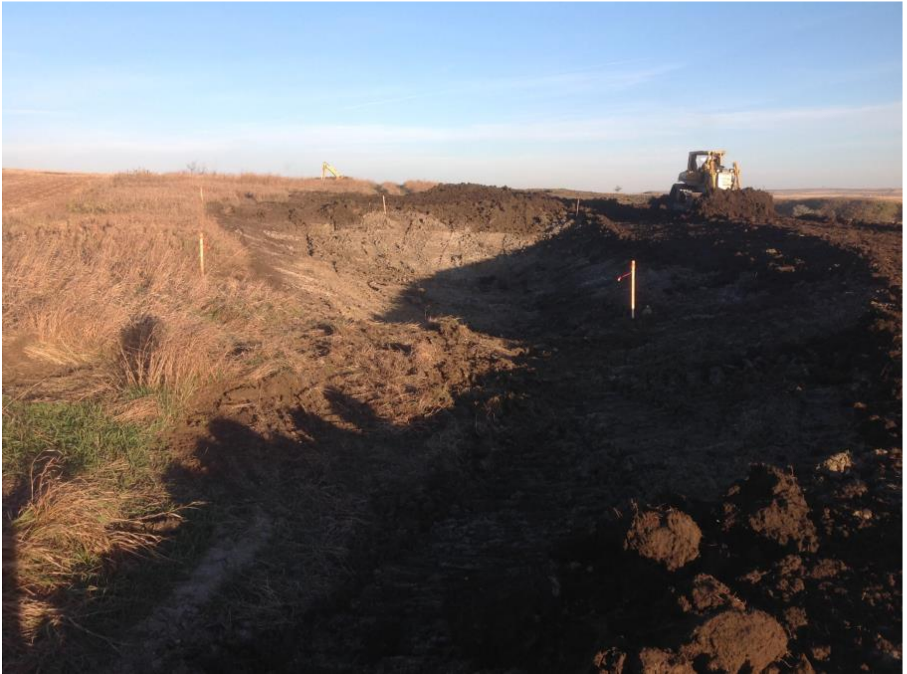
Construction of Small Wetland Sump to Help Control Surface Water Runoff
