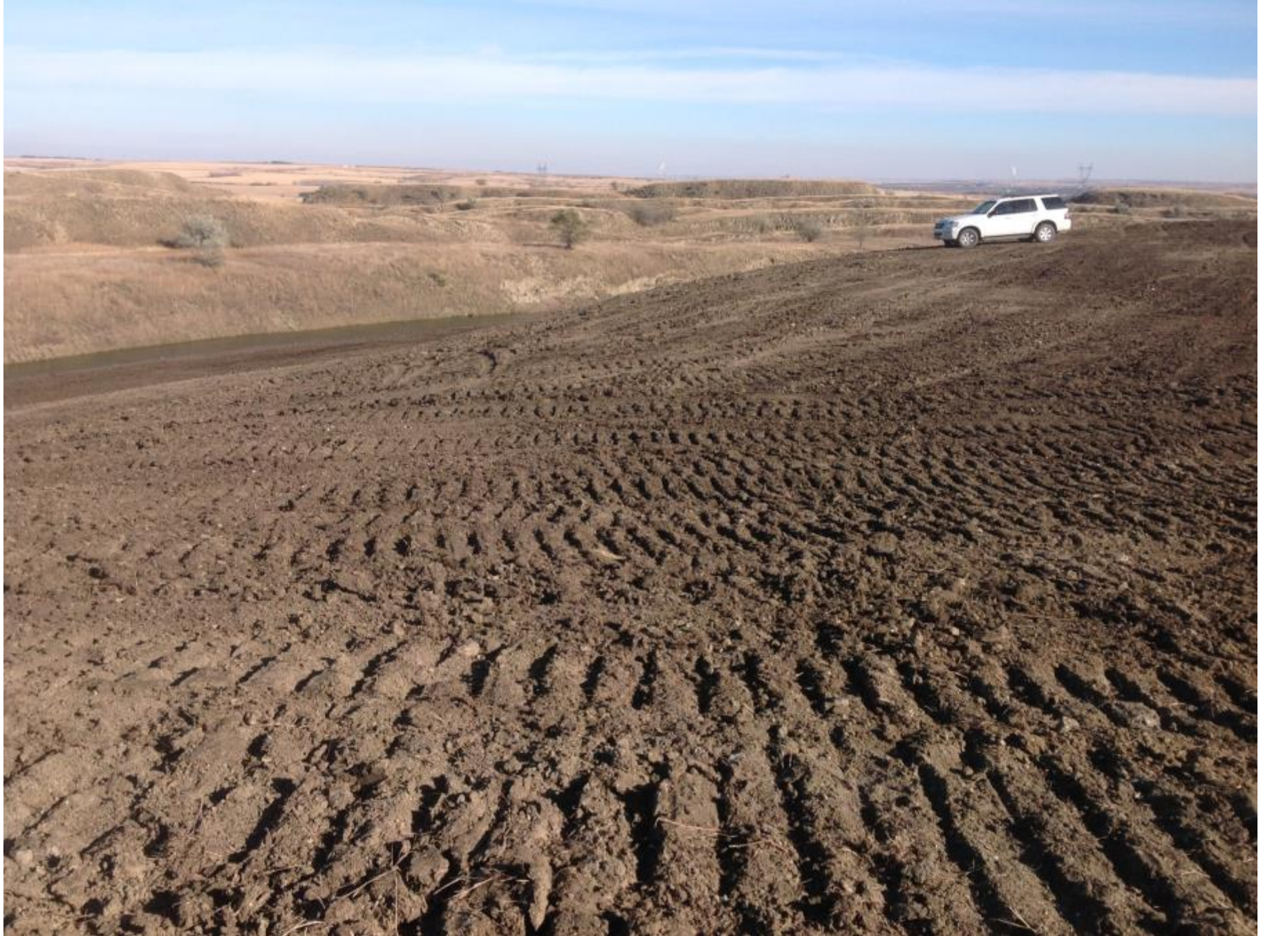
Post Reclamation Slope Following Topsoil Respread Operations
