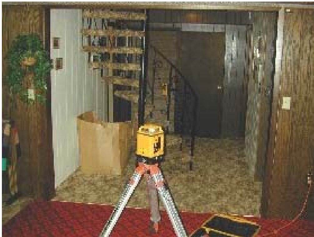
Figure 4: Laser level and target used to monitor structural movement in Thielman's basement.
