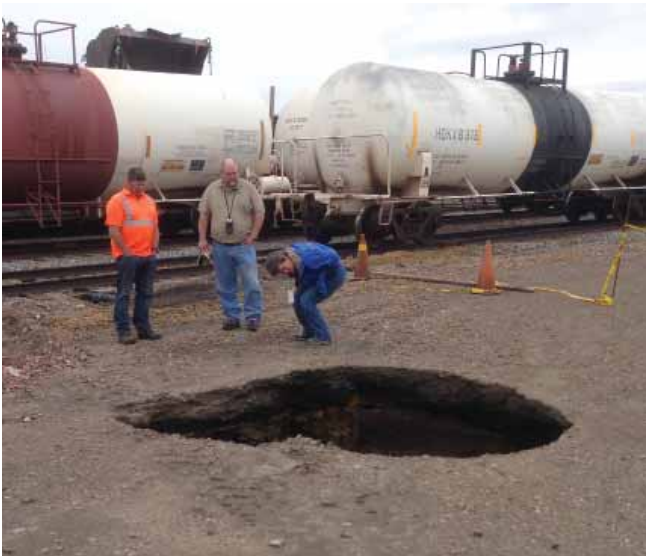
Sinkhole southeast of Dickinson
