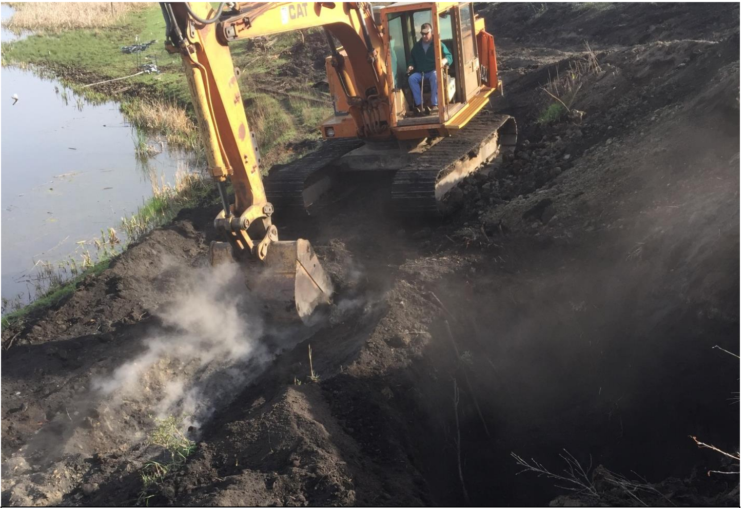
Above: Moving burning materials into pit, where it was mixed with wet clay and buried. Photo date June 4, 2015
