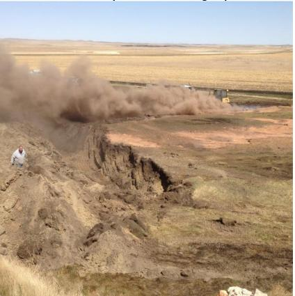
Work began on April 22, 2015. This shows a Cat D6K Bulldozer pushing burning coal screenings into a burial pit. The burning materials were mixed with wet clay and buried. When these materials were exposed to air, they began to burn at temperatures over 900°F and the smoke could be seen from miles away.
