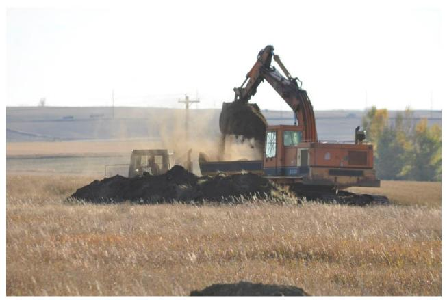
Approximately 13 sinkholes were filled on property owned by James Kimball a mile south of Noonan on October 12-18. This shows topsoil removal and excavation of fill dirt from a borrow area at the west end of the site.
