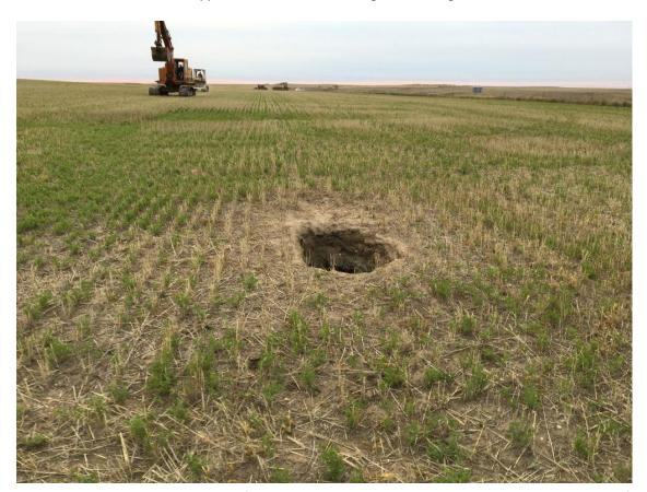
Three sinkholes and a couple settled areas were filled at the Hanks site on October 11-12. The approximate cost for this work was \$1875. About twenty dangerous sinkholes have been filled on this field over the past ten years.
