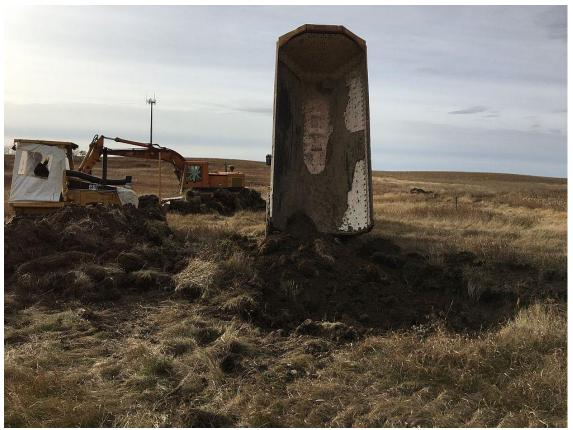
Eight dangerous sinkholes were filled at the New Salem Site on October 31, with about twelve truckloads of dirt. The contract cost for this work was \$2093.75. More than 50 sinkholes have been filled at this site since 2005.
