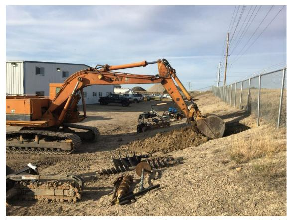
This sinkhole and another one, on nearby commercial property owned by Sand Draw, LLC, were excavated and filled October 10-11, 2017. The approximate cost for this work was \$1875. An AML drilling and grouting project is planned here for 2018.
