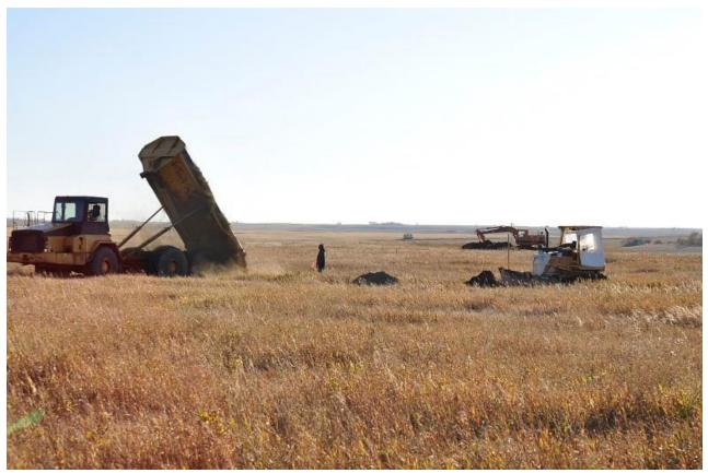
This shows an off-road truck dumping dirt into a sinkhole, while a bulldozer is leveling dirt on another sinkhole. The excavator in the background is excavating fill dirt from the borrow area. The approximate cost of sinkhole filling at this site was \$2870.
