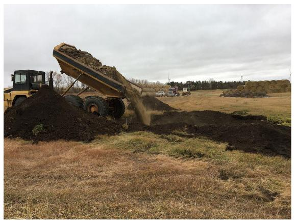
This shows the same sinkhole while it was being filled. Seven truckloads of dirt were needed to fill it. Then topsoil was respread and it was tilled and seeded. Twenty two sinkholes were filled near Wilton, October 24-26, and the contract cost was \$4182.50.
