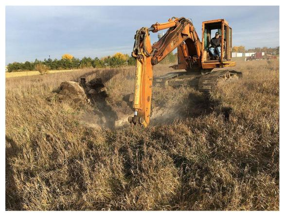
This shows the excavation of a sinkhole south of Garrison. It was about 8 feet in diameter and 10 feet deep. Thirteen sinkholes were filled at this site on October 19, 2017, and the contract cost for this work was \$1995.
