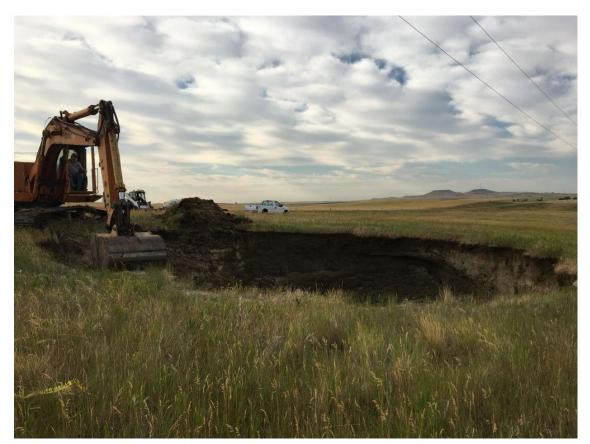
Work began on the 2017-2018 Sinkhole Filling AML Project on July 21, 2017, about 4 miles north of Bowman. This sinkhole was about 30 feet long, 20 feet wide and 18 feet deep. It was located on property owned by the City of Bowman (see cover photo).
