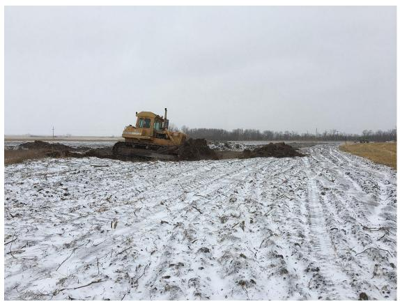
This shows the contractor saving topsoil from around a sinkhole during a snowstorm on November 3. Approximately 1000 cubic yards of dirt were moved to fill the 31 sinkholes at a cost of \$9750.
