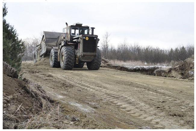
This hole was 45 feet long, 18 feet wide and 15 feet deep and required about 25 scraper loads of dirt. In 2017, seventy dangerous sinkholes were filled near Beulah at a contract cost of \$73,111.75. Over the past ten years, about 410 dangerous sinkholes have been filled near Beulah at an approximate cost of \$350,000.
