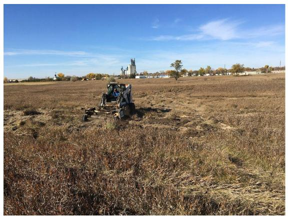
Topsoil was removed before filling each sinkhole and replaced after the sinkhole was filled with dirt. After respreading topsoil, the contractor was required to till each disturbed area and seed it to a native grass seed mixture.
