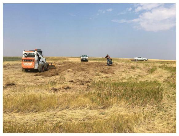
This shows the contractor tilling and seeding the same area after the sinkhole was filled. Approximately 60 truckloads of waste concrete and dirt were needed to fill this large and dangerous sinkhole. The contract cost for this work was \$6237.50.
