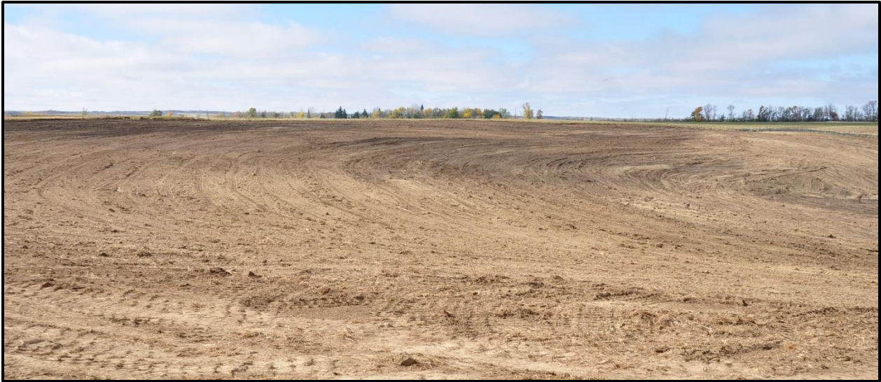
Site 3 Final Grade
