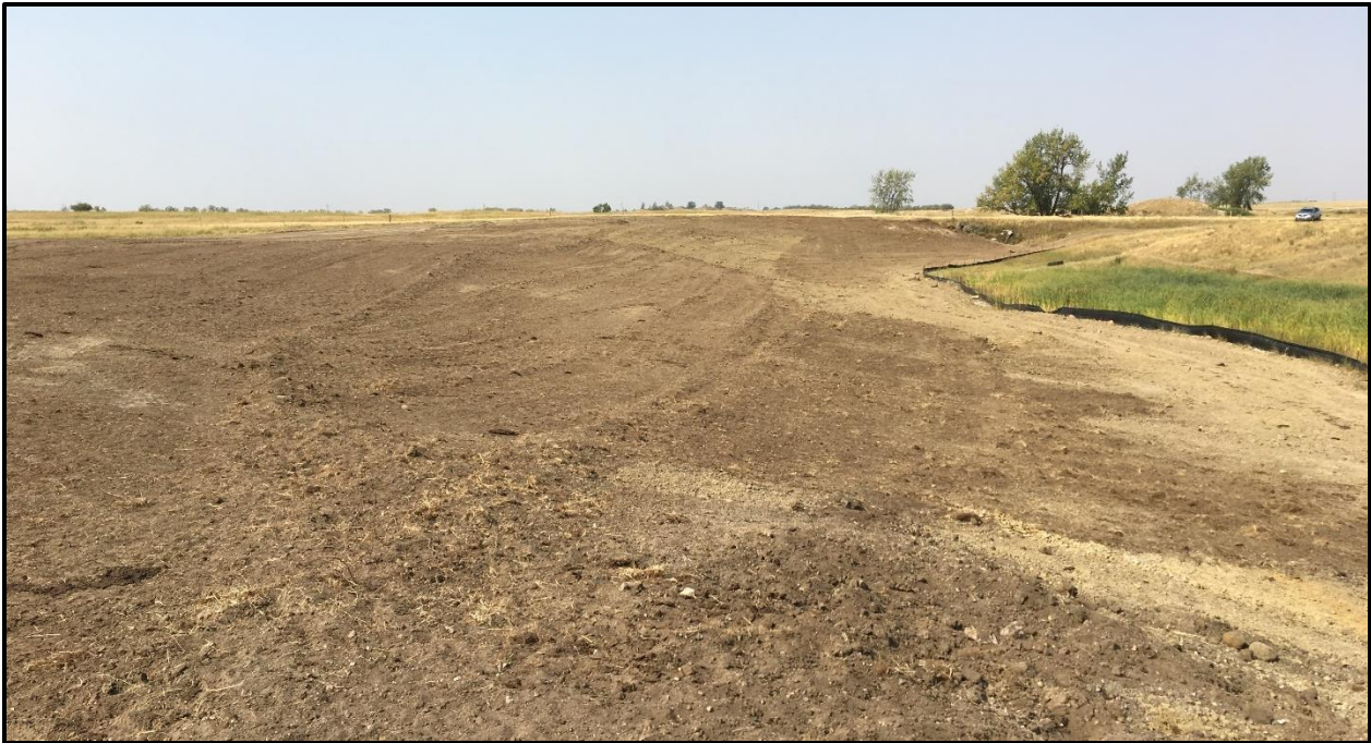
Site 2 Final Grade
