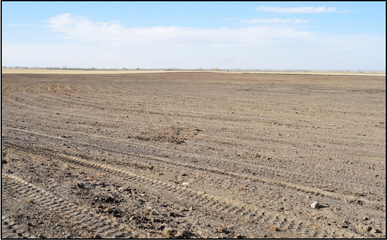
Site 1 Final Grade
