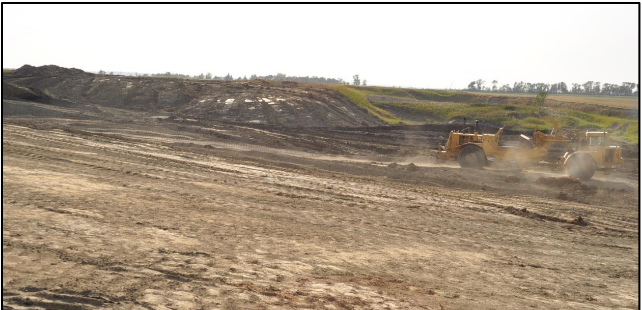
Site 3 Topsoil Salvage
