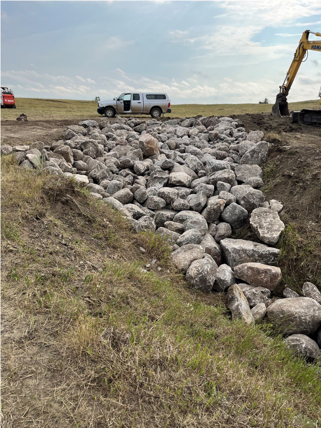
Figure 11: A large erosion gully was graded and stabilized with rip rap.
