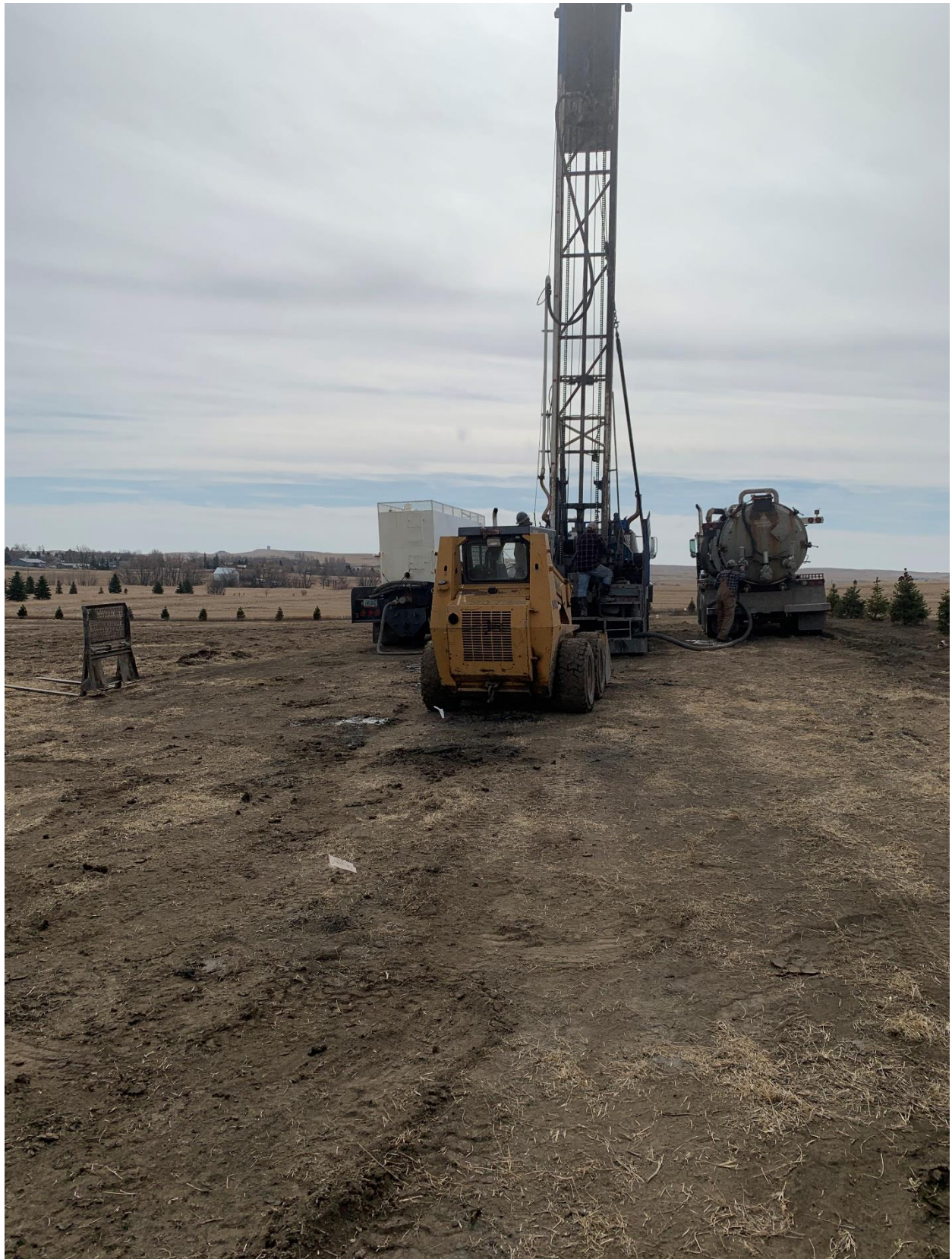
Figure 5: The vacuum truck (on the right) is capturing drill cuttings and water produced by drilling.
