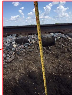
Shows depth of hole created by collapsed drainage culvert.
