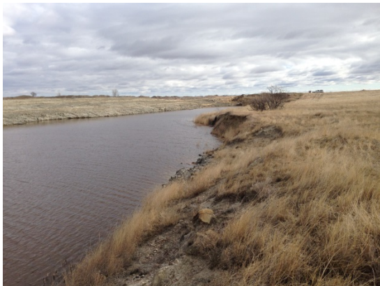
Photo 2: Newly seeded & sloped highwall (far bank) and developed water resource.
