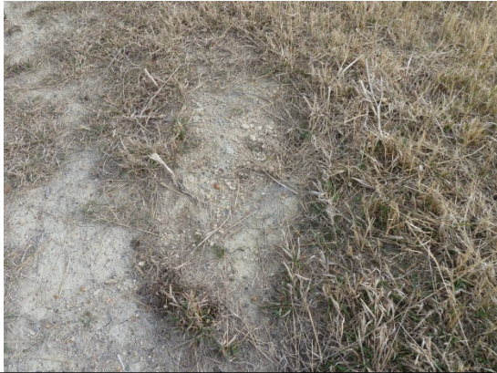
Photo 7: Scranton Site. Properly filled borehole east of 133 rd Ave. SW.
